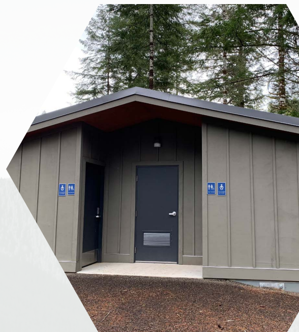
New Restroom Facilities
